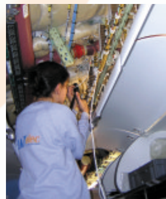
Intervention cabine Cabin outfitting
